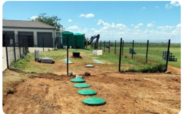
2023 - 50% capacity added without changing the initial infrastructure.
