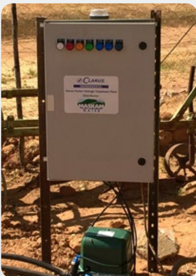
13:30 - Fusion electrical panel (with EWS) and air pump installed.
