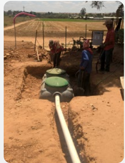
12:38 - Filled with water and backfill underway
