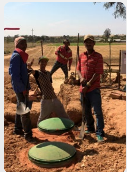
15:05 - Installation complete. Maskam Fusion® fully operational
