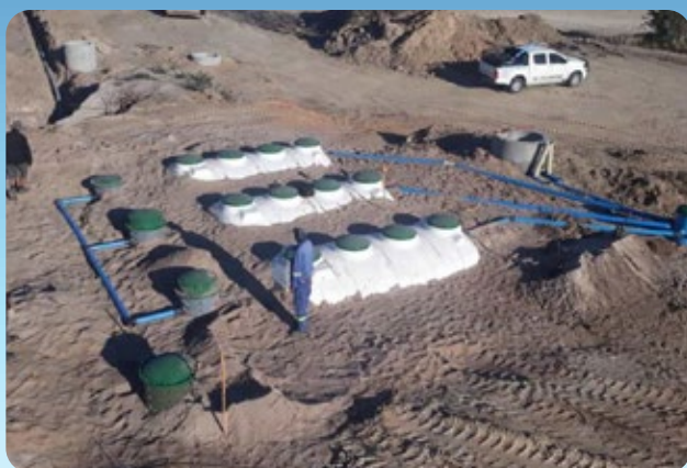
Equal flow splitter (can accommodate 6 plants)
