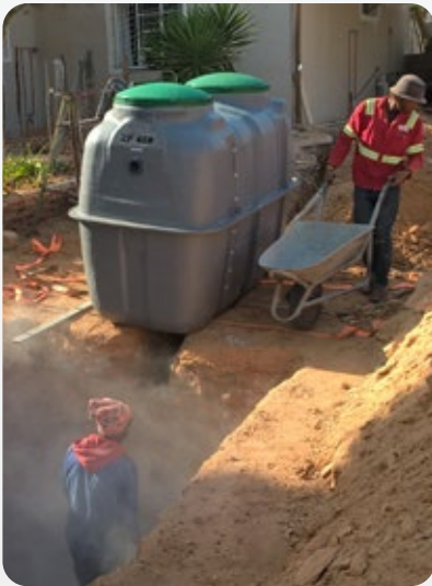
08:38 - Fusion® delivered and preparation for placement underway.
