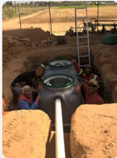
09:58 - Fusion® in place and inlet pipe connected.
