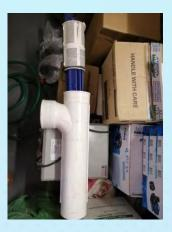
**The Second Manhole** is for the UV and needs to be checked ones every six months and if faulty needs replacement (UV Tech 75 Watt UV Lamp).
