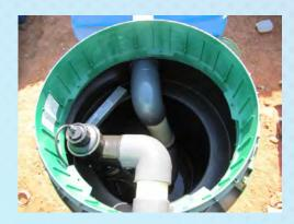
**The Third Manhole** is the 6 000 Litre Storage tank and needs to be checked every month to make sure that the 40 Litre /m Fine Bubble Blower blows air into the system, it can also be checked at the Control panel if the Air pomp is operational.
