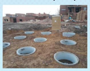
**The first Manhole** is inflow from the splitter box to the 1000 Litre Pre Tank equipped with a Inline Filter on the outlet of that tank, this Filter needs to be cleaned once a month for the start to determine frequency of cleaning.
